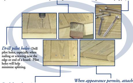
Deck board spacing- During construction, should the wood become wet, butt deck boards together. As drying occurs, some shrinkage can be expected. If the wood is dry, allowing for shrinkage is not necessary.
