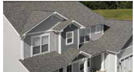
ROOFING AND VENTILATION
